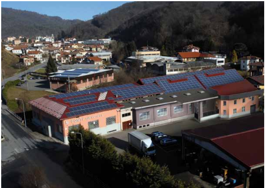
→ Conti manufacturing facilities and foundry
